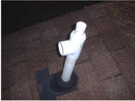
Before the adapter was placed on the vent pipe I smeared a bit of light grease on the vent pipe. This will allow for easy disassembly should the need arise. Finally, what does the whole thing look like installed? Here's one that installed on my roof. No expensive mounts or
