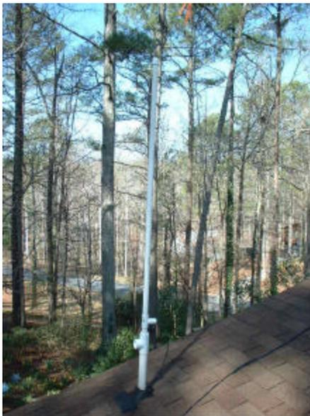
hardware needed. Just the rear deal. Again, don't glue any downward facing joint. The glue is used not only to hold parts together but to act as a weather seal. If a joint faces down then it's not likely going to provide a path for moisture to invade a space.
