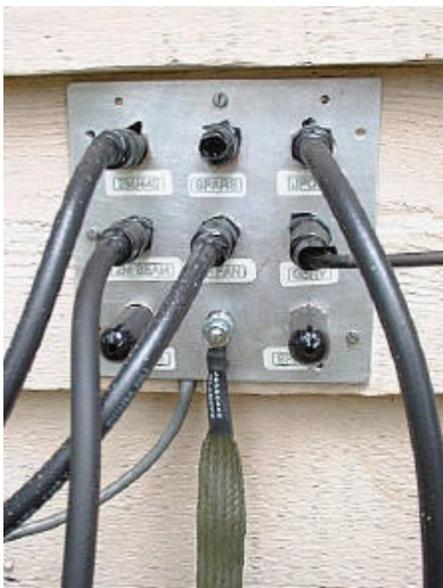
The outside bulkhead grounding arrangement has the other side of the 1/4 inch bolt going through the bulkhead to which a 1 inch braid is connected going
