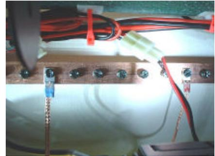
threaded them with a 10-32 tap for common ground screws available at any Home Depot. I might have gone to an electrical supply shop and bought a regular buss bar. Where's the fun in that anyway? Also, there's no promise that it would match up with how I wanted to mount it to the shelf supports. Besides, this was cheaper and it was late at night when I did this part of the job.
