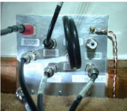
At the top left is the beam antenna rotor control cable. At the upper right is the ground cable from the radio shelves. This stranded cable doesn't go into the floor but I routed it along the mop board and then up to the shelves. All the metal shelving supports are grounded together. More about them later.
